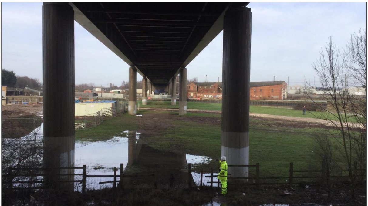
Figure 5-1 – Photograph taken during Atkins Site Walkover beneath A46 viaduct over River Trent / East Coast Main Line
