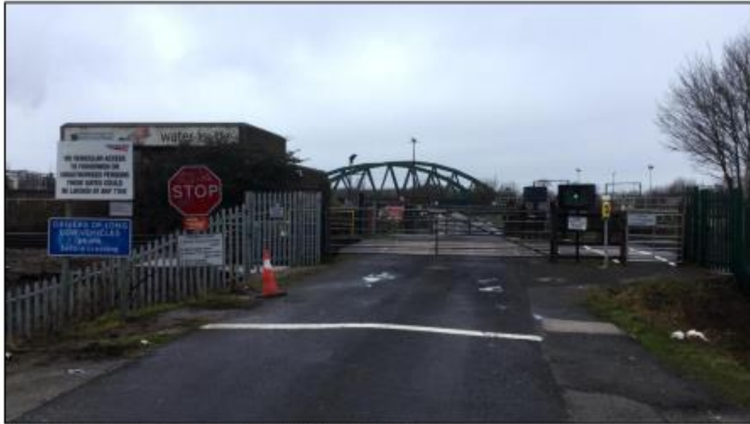
Figure 20 - Level crossing access to sewage works. Looking north,
