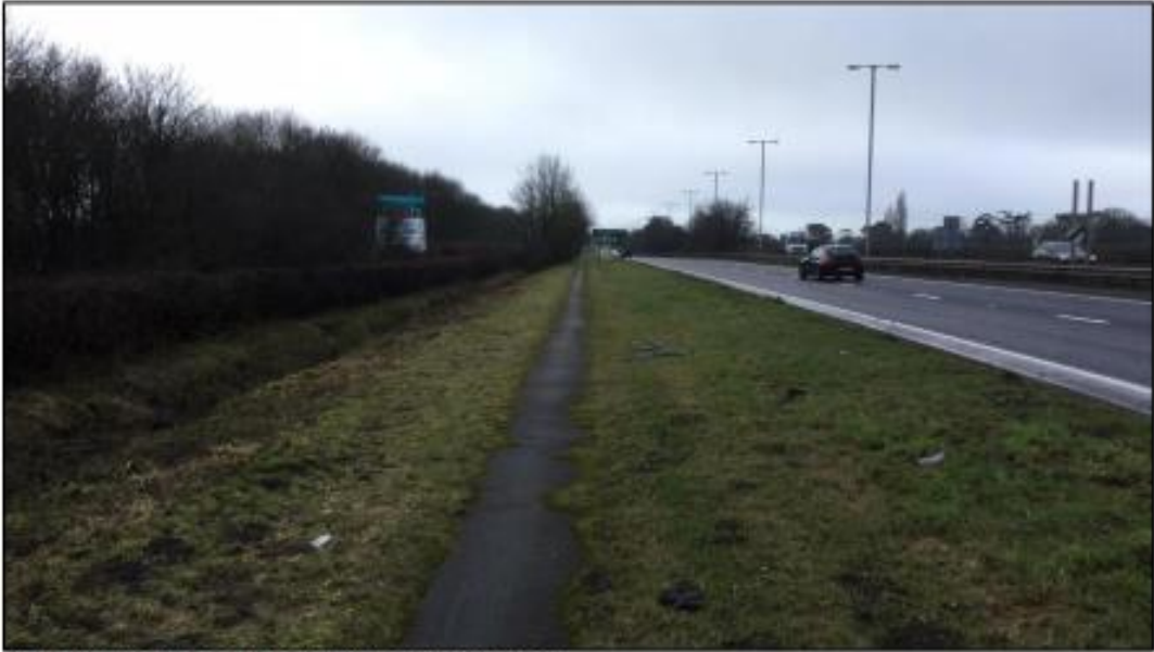
Figure 32 - Looking south from Winthorpe Roundabout.
