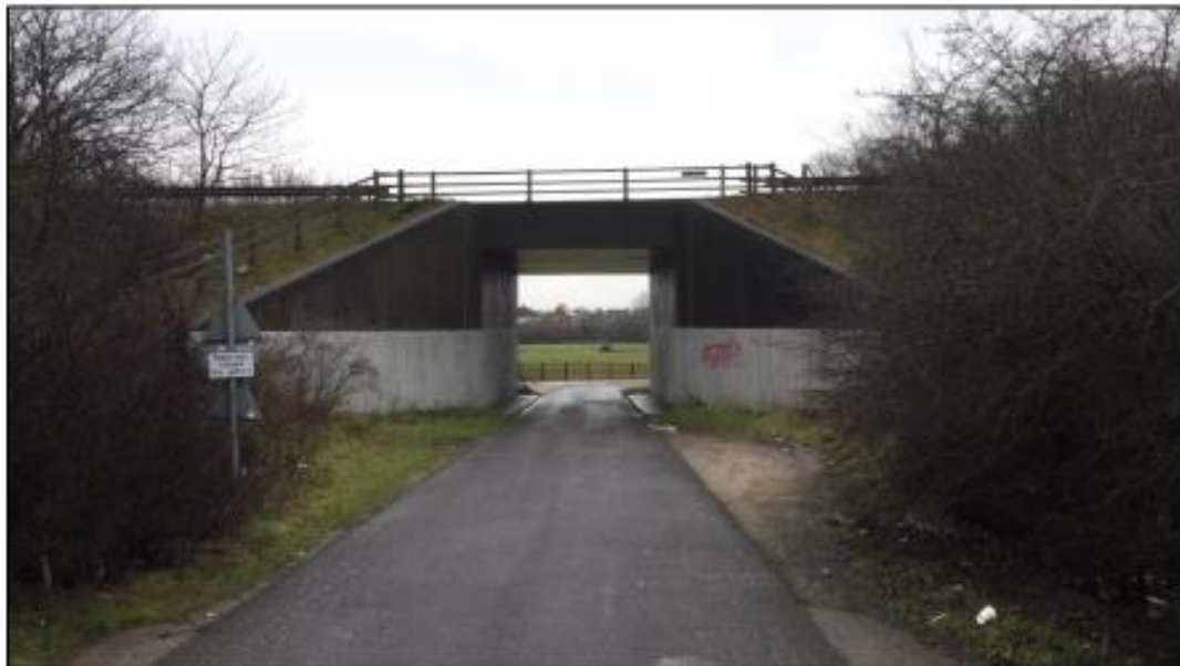
Figure 21 - A46 underpass (access to sewage works)
