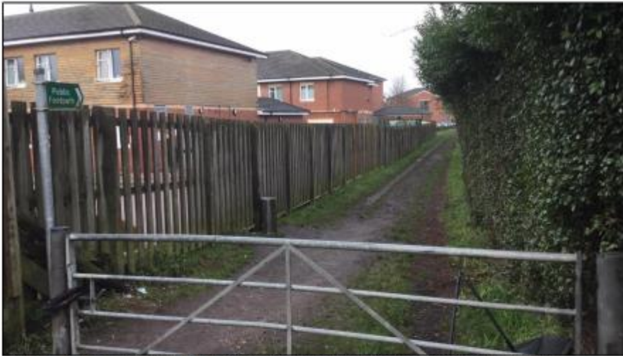
Figure 4 – Access track leading to to area beneath viaduct over River Trent, from B6166, Farndon.
