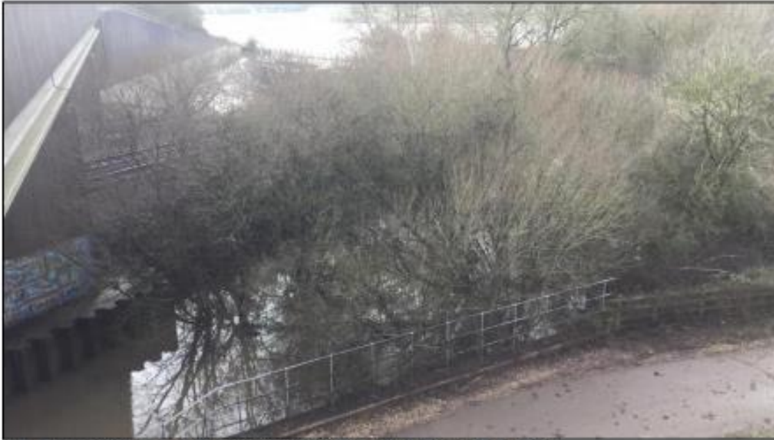
Figure 10 – Looking south, bridge NOB1/53A over Nottingham to Lincoln railway.
