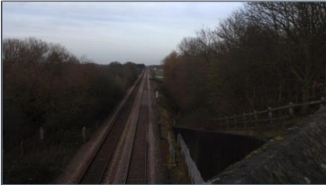
Figure 16 - Bridge 61A over Nottingham to Lincoln railway line looking north towards Newark Crossing.
