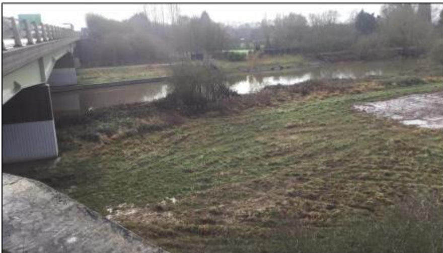
Figure 5 – Looking south over River Trent from viaduct wing wall, Farndon.
