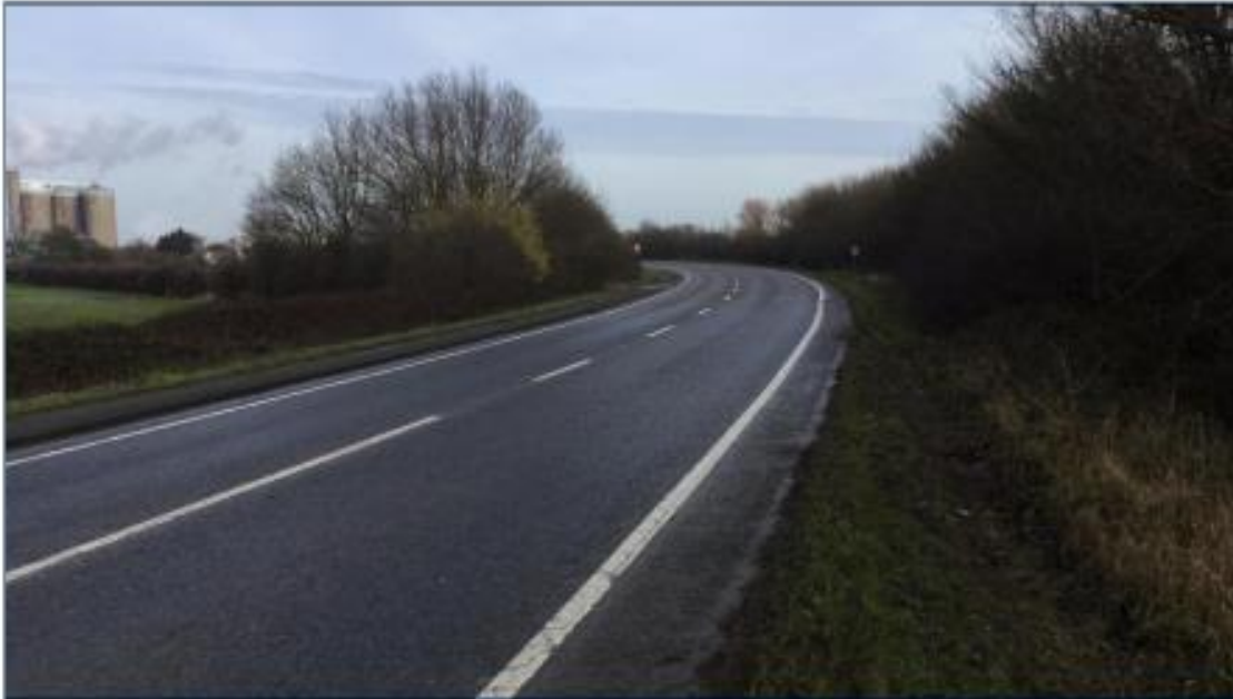
Figure 14 - A617 looking east towards Cattle Market Roundabout and Sugar Works
