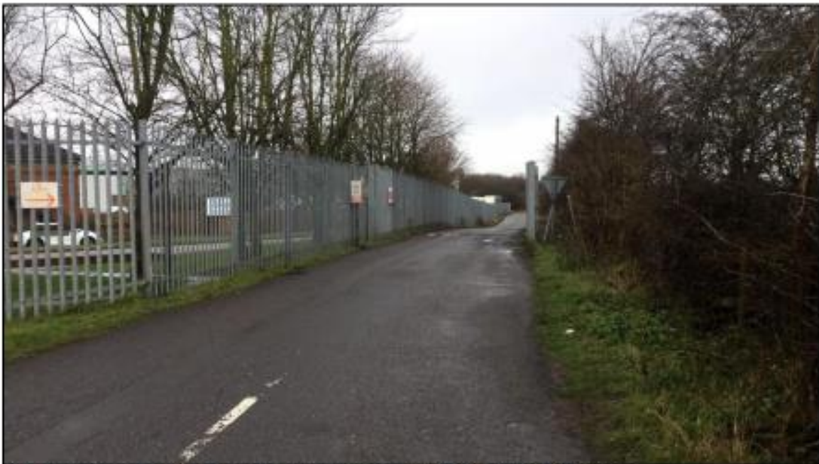
Figure 23 - Access road to sewage works (public footpath) leading from Quibell's Lane
