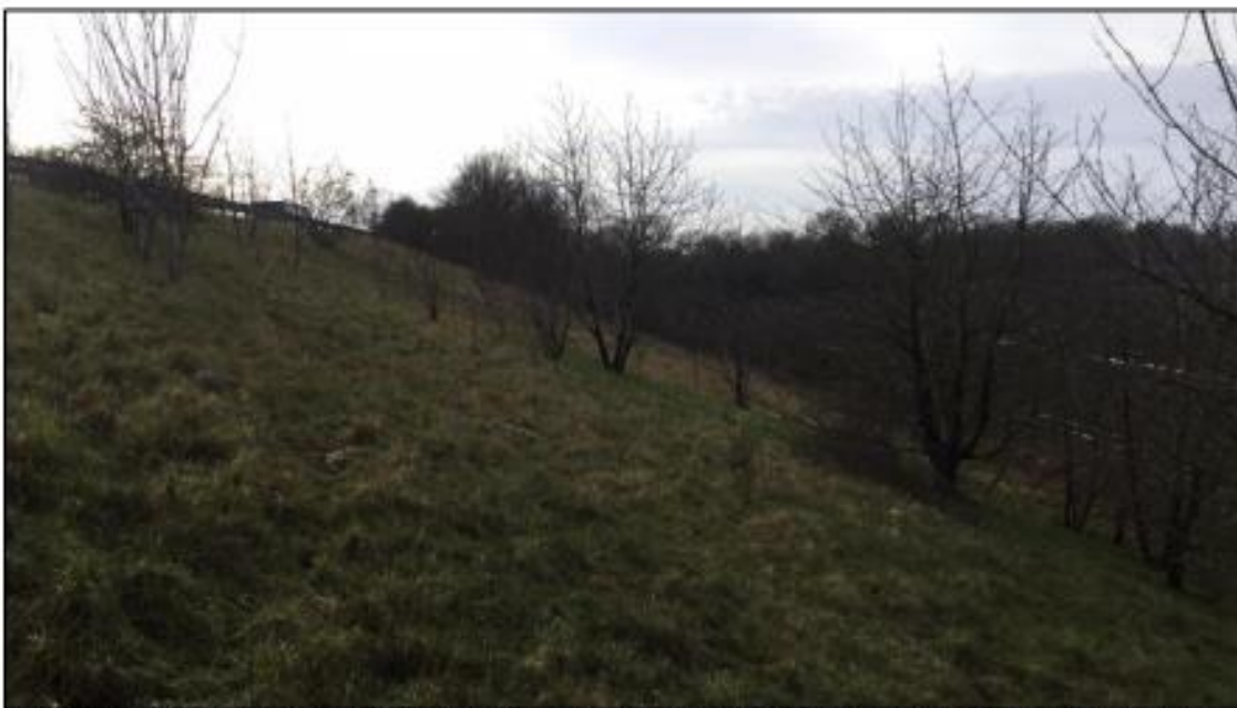
Figure 11 – Typical view of earthworks between Cattle Market roundabout and Nottingham to Lincoln railway, looking south.
