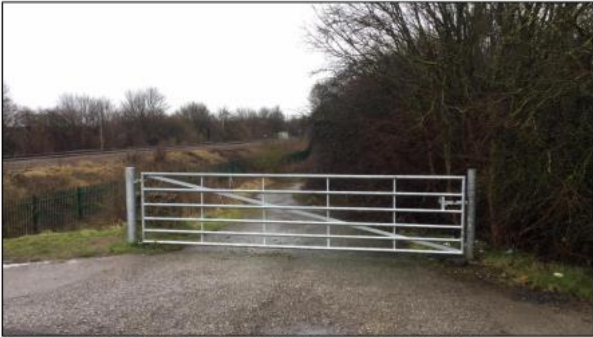
Figure 22 - Access point adjacent to level crossing (sewage works access). Looking north.
