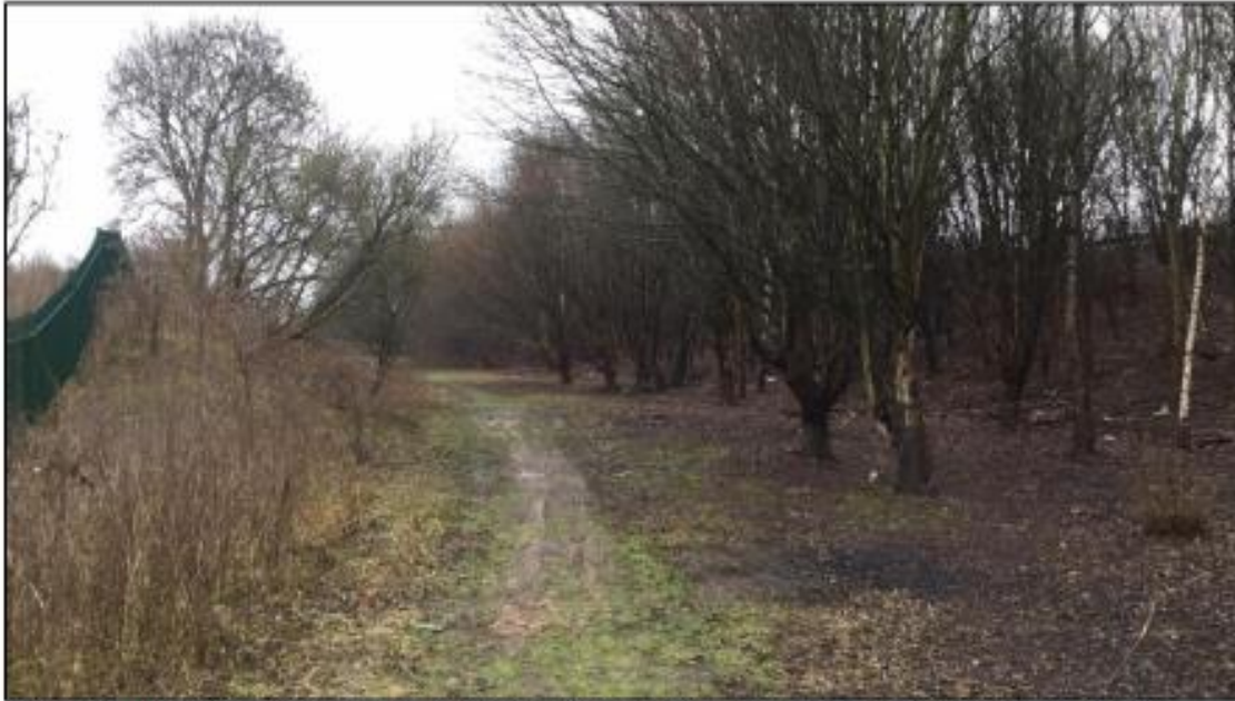
Figure 24 - Wooded earthwork slopes between A46 and Nottingham to Lincoln railway line, looking north. Adjacent to sewage works.
