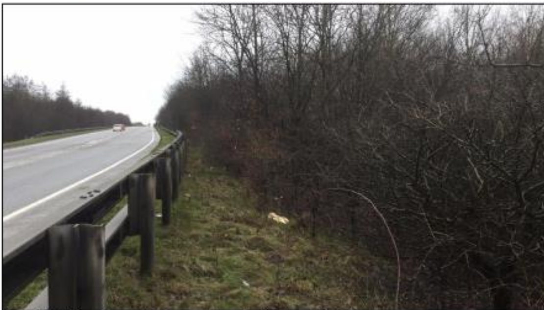
Figure 25 - A46 carriageway looking south towards viaduct over River Trent.
