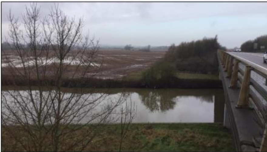
Figure 2 – Looking north, A46 viaduct over River Trent at Farnon end of the scheme.
