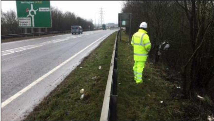
Figure 1 – Looking south towards Farnon Roundabout at southern end of scheme.
